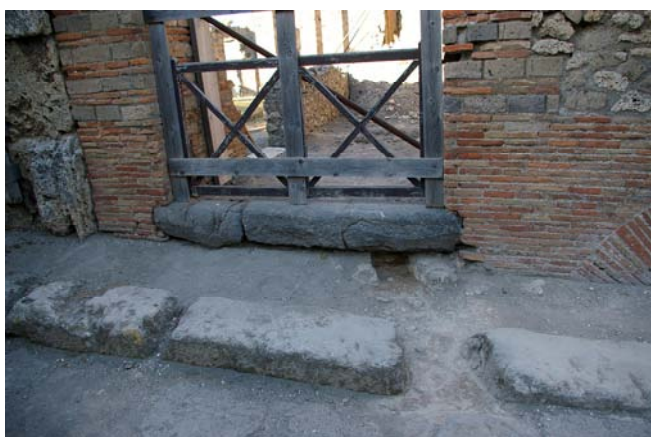
Fig. 9. Pompeii VI 8, 20-21.2, back entrance 2: drain from fullonica.
